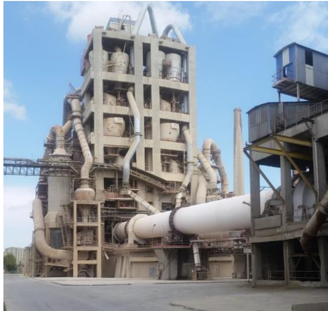
Figure 3. Kiln and cyclone pre-heaters view at SECIL plant in Maceira Liz
